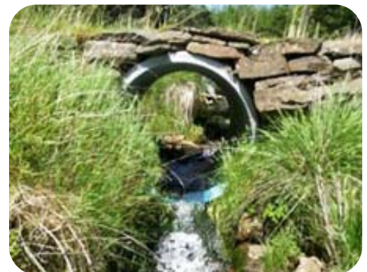
Culvert (Afan river, United Kingdom). J. Jones (2019)
