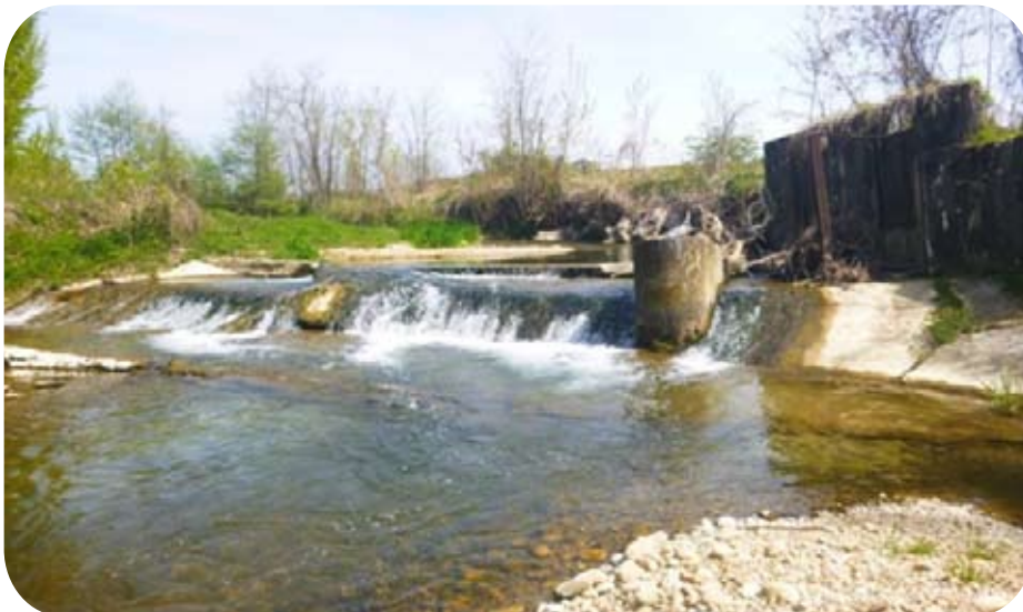
Last weir before removal in the Herbasse river. (Photo credit: SIABH)
