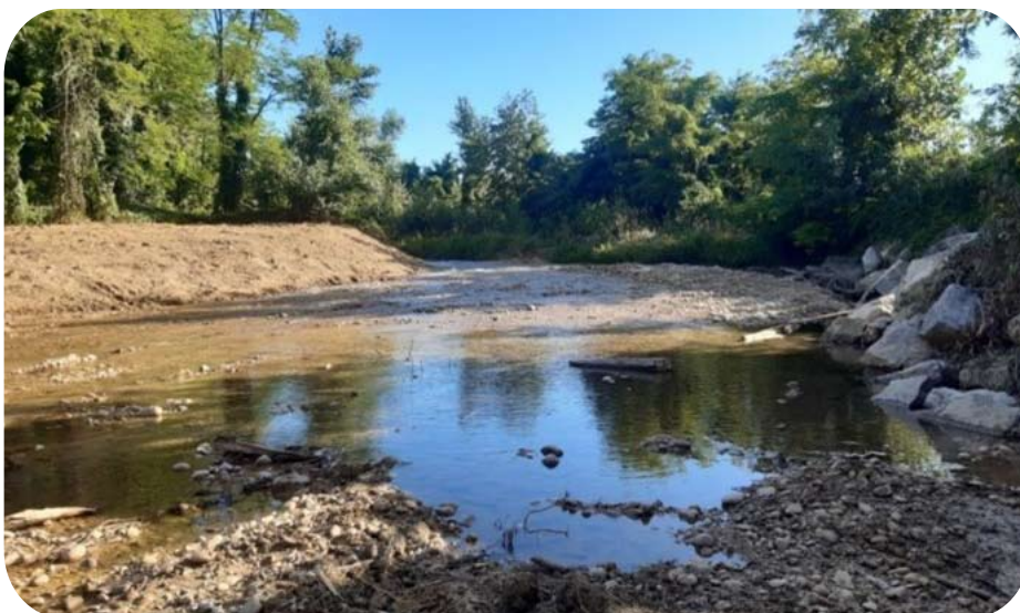
After last weir removed in the Herbasse river. (Photo credit: SIABH)
