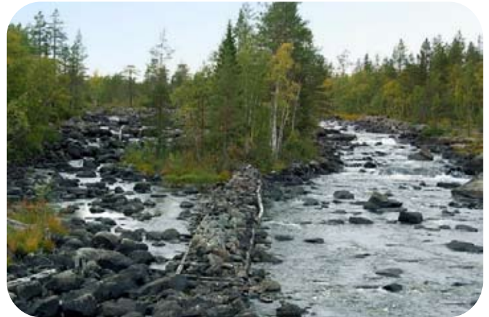
A rapid in Varjisån, a tributary in the Pite River system in northern Sweden with stone walls blocking the flow in a side channel facilitating timber floating. (Photo credit: Roland Jansson.)
