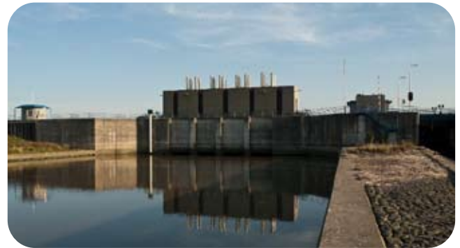
Tidal sluice gate (Netherlands). J. Van Deelen (2017)
